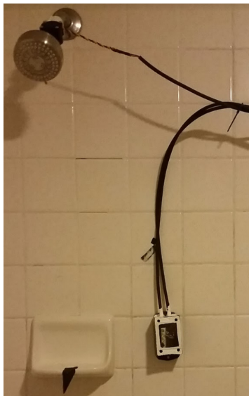
Figure 2: Flowmeter installed on showerhead
