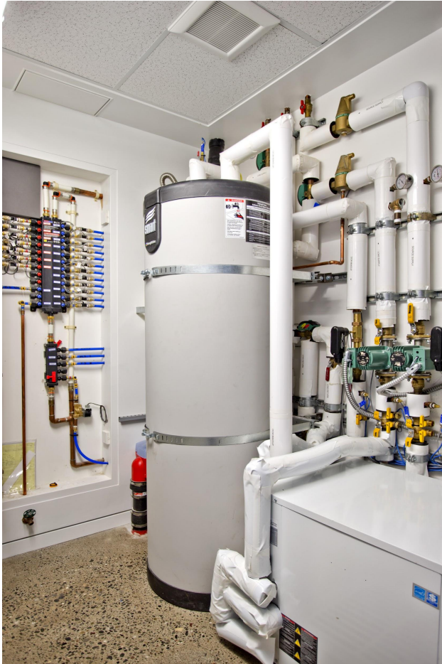
Figure: (Left) Mechanical room, including (from left to right) manifolded domestic hot and cold water distribution system, domestic hot water storage, hydronic plumbing, and water-to-water heat pump. (Right) Greatroom, including radiant slab on the first floor, and radiant ceiling (with ceiling fans) on the second floor.
